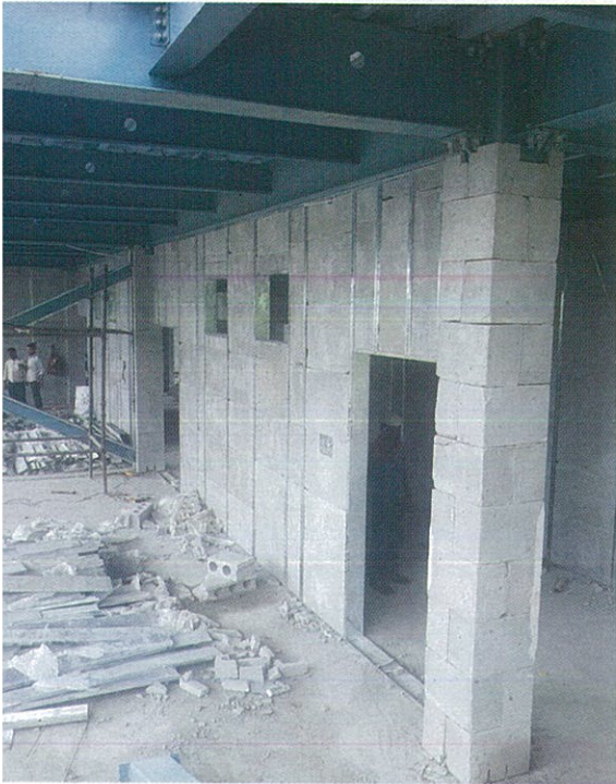
Internal Beam & Joist
