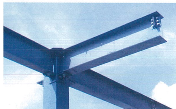
Column Beam Joint
